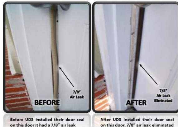
AIR LEAK LEFT SIDE OF THE DOOR
